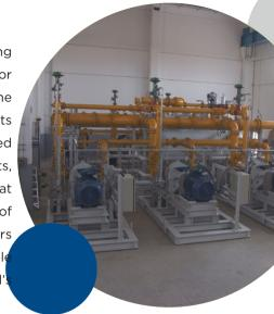
Designed, manufactured, tested, and delivered in 2012 the 'Cobalt' system consisted of three GARO C 80 2.5 Ti liquid ring compressors. The package was commissioned in 2014 during a planned maintenance shutdown.
